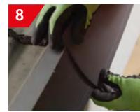
The second verge can easily be positioned by locating the front edge of the verge over the two notches on the installed verge, and sliding up until it meets the leading edge of the tile.
