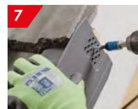
Once in position the verge unit can be screw fixed into the end of the batten using 40 x 3.5mm stainless steel screws.
