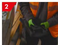
Fix the eaves closure -Next, you will need to fix the Eaves starter. Establish the position of the starter unit by making a mark by positioning it inside a verge unit and placing it in position, flat on top of the tile. Now remove the eaves starter prior to fixing.
