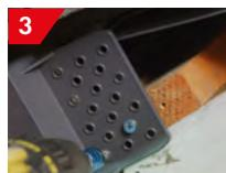
The eaves starter unit should be twice fixed to the end of the fascia board, brickwork or timber tilt fillet.
