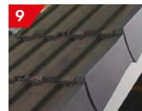
This process can now be repeated, ensuring each verge unit engages with the one below, so a verge unit covers the end of every course of tiles.
