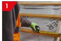
Extend the tiling batten -Once the roof has been felted, you will need to install the tiling battens, ensuring they are extended 35mm beyond the gable wall, barge board or render. This will allow for screw fixing the verge.
