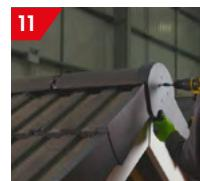
To finish, screw fix the Ridge End Cap to the ridge batten, securing it in place and completing the Ambi Dry Verge system. The ridge system will need to be installed prior to fixing this. If required a small slot can easily be made on each side of the end cap so it sits over the upstand of the verge unit.
