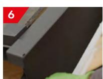
Fit the first verge section making sure that it is located firmly onto the eaves starter.
