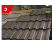
The roof is now ready for tiling in the normal way, ensuring the tiles finish flush with the end of the batten.
