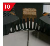
Insert Ridge Closer into the last unit - When we reach the top or apex of the roof, we can close this area off by using the ridge comb that is supplied as part of the eave and ridge kit. The teeth of the comb sit over the bottom edge of the verge unit where it will be held in place. If using a dry ridge system the ridge roll can be extended over, tucked back up and stuck to the underside to offer additional protection.
