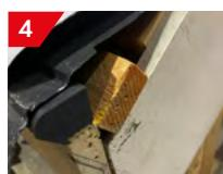
An additional batten behind the fascia board can also be used if required to ensure a suitable fixing point - this should be securely fixed to the rafters.
